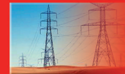
High & Medium voltage lines
